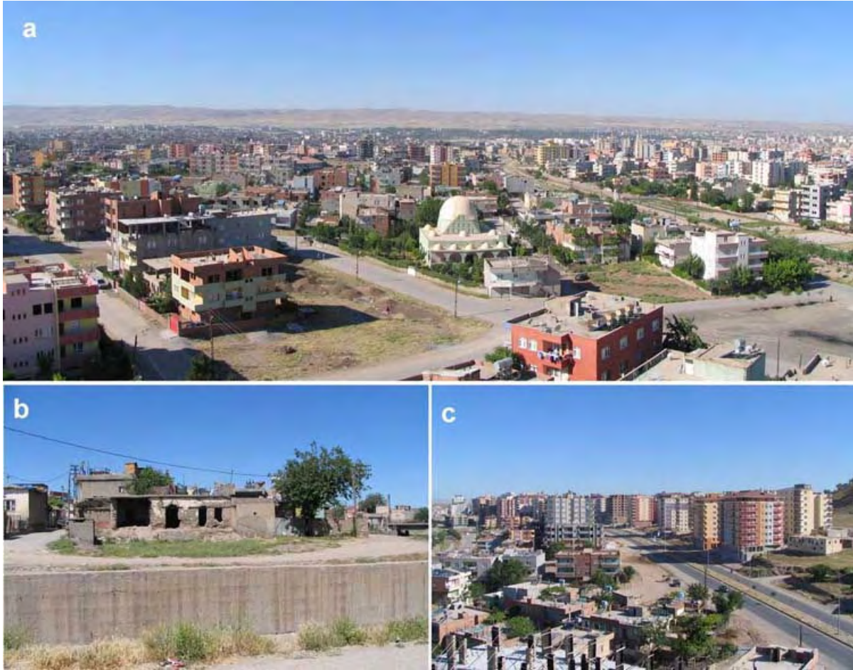
Figure 8: Dwelling types in different districts of the city center of Batman. a) Multi-storey buildings constructed in the north of the city in recent years and single-storey dwellings in the south. b) Dwellings constructed illegally and severely damaged in the flood disaster of 2006. c) Modern buildings constructed in the northern part of the city in recent years.
