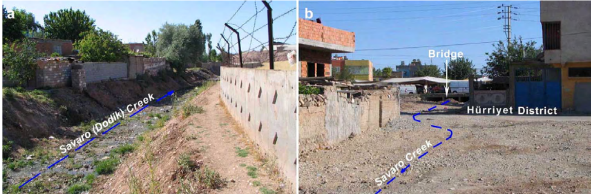
Figure 13. Savaro (Dodik) Creek affecting the southern part of Batman city. It is seen that the stream bed is wide at the entrance of the city but appears narrow in the district of Hürriyet. a) Wide bed of Savaro Creek at the entrance of the city. b) Status of Savaro Creek in the district of Hürriyet.
