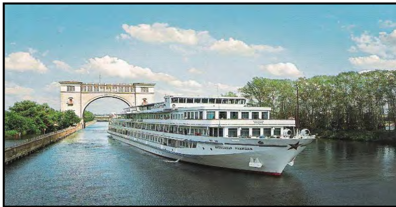
Photo 1: An Example of Lock Elevation from Uglich
