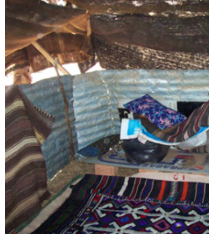
Photos 7-8: Usage of Nylon Sacks and Corrugated Tins Instead of Putte Mats (Photos 7-8: Ayşegül KOYUNCU Archives, İzmir/2008)
